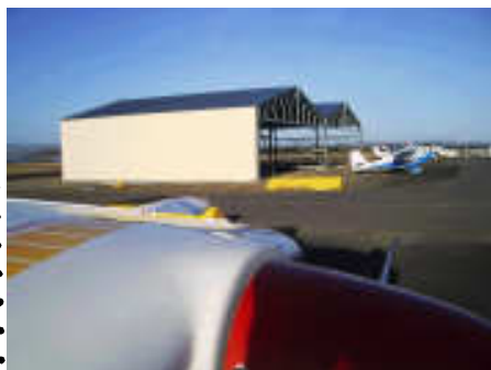
Cladding & roof goes on the new hangars
