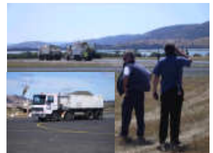
Don Wells & Martin Scott sealing Rwy 32
